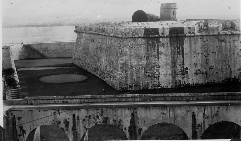
Remains of old lighthouse atop Morro Castle, San Juan, Porto Rico.
