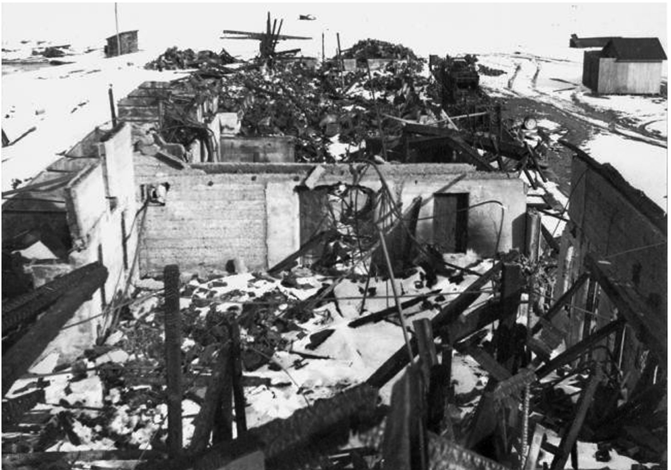
Structural fire destroyed the Orrtanna Canning Company property on December 3, 1942. The company had no buildings to store finished goods and no cash reserves.
