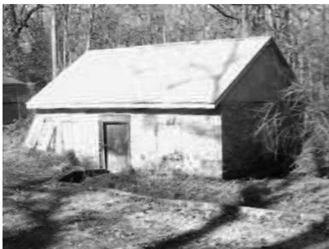
This two-room stone structure springhouse was built by Ludwig and Margareta Lindemuth at 508 Pinkerton Road, Mount Joy. It was built on top of an old quarry with a solid stone foundation. Thus, the walls stand firm by an extremely active spring. In recent years, it was used as a fish hatchery. (Nelson and Mary Ginder, 2020)
