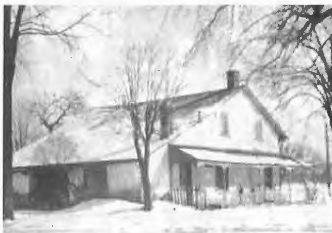
The Baker homestead near Saint Thomas, Ontario, built by William Baker (no. 24) about 1850. The house was constructed by placing clay, straw, and water in a pit and then driving oxen through the pit to mix them. The house walls were erected by pouring the mixture into forms and then allowing it to dry. The eighteen-inch-thick walls were raised in three-foot increments. The house is still occupied by descendants.
